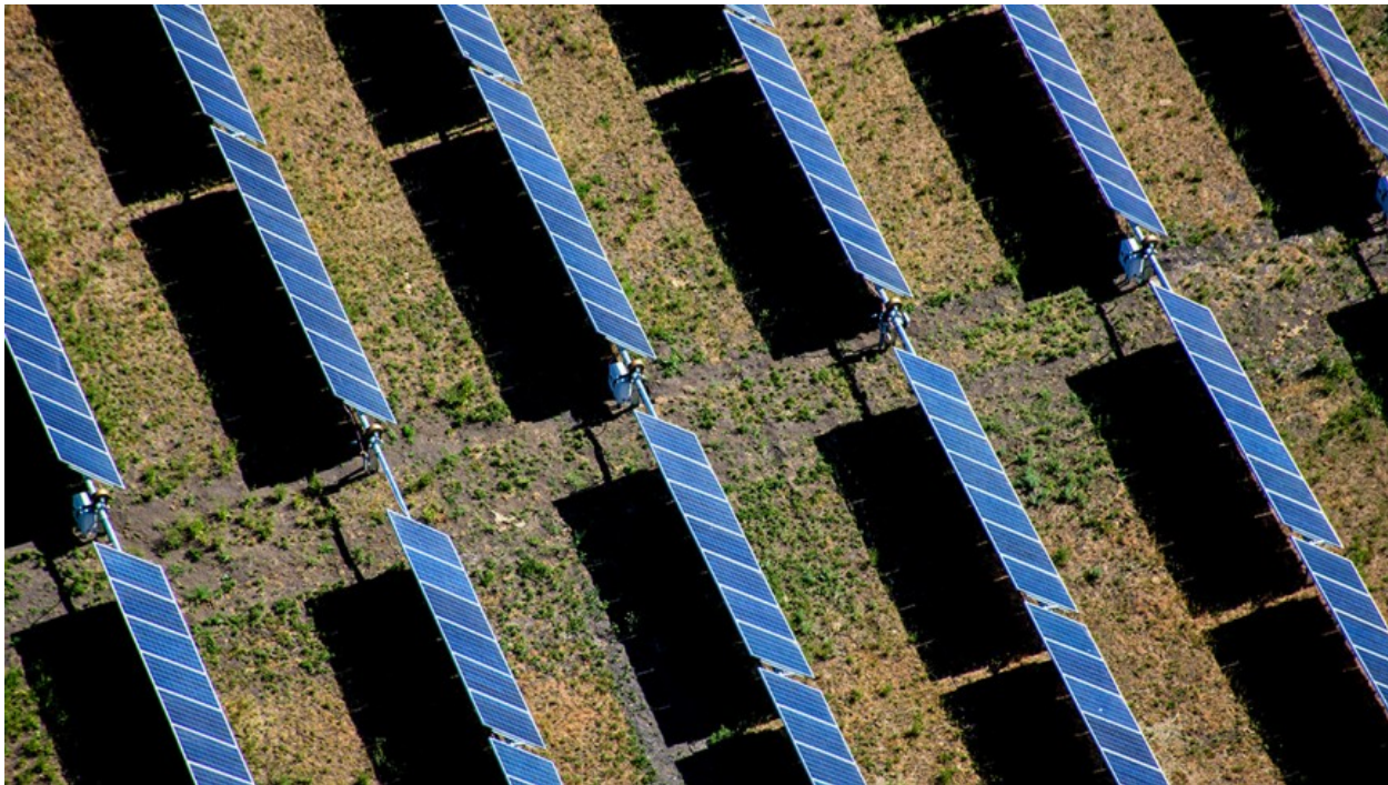
Figure C. Rows are spaced 15 to 20 feet apart, as required to address slope concerns.
